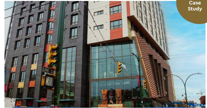
The new First United Building, set to open its doors in spring 2026, will provide critical services and support to the local community
