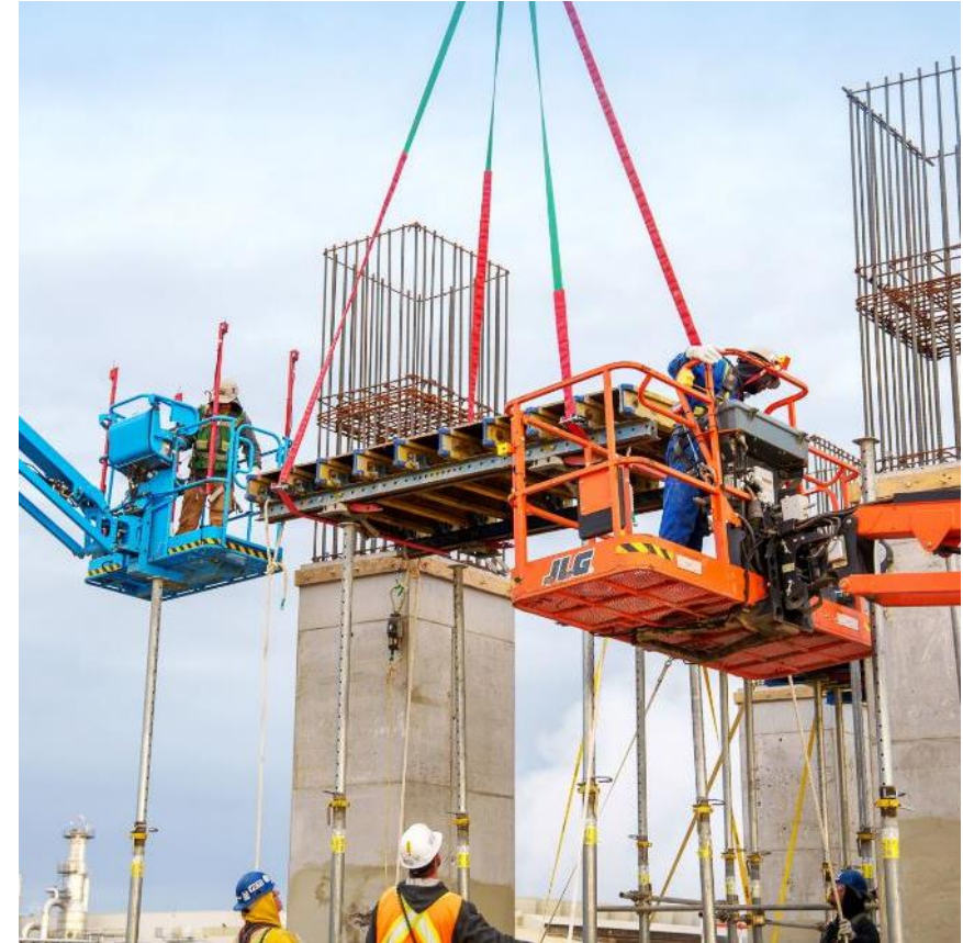
DOW FORT SASKATCHEWAN PATH2ZERO EXPANSION PROJECT // ALBERTA, CANADA
