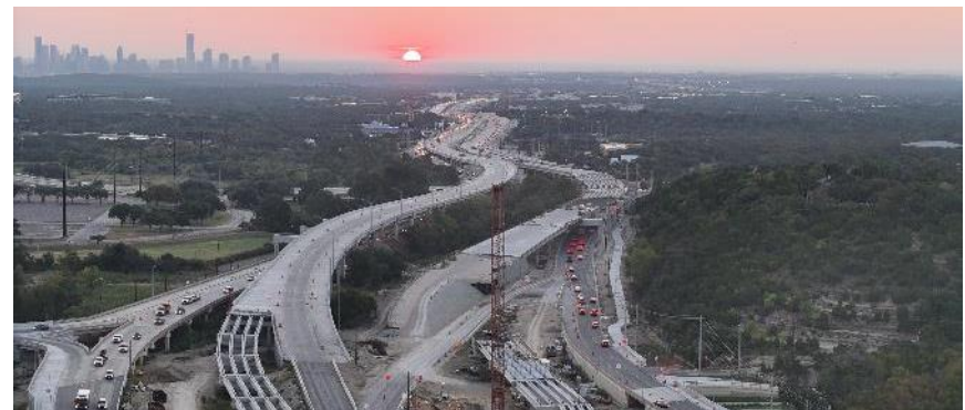
OAK HILL PARKWAY PROJECT // TEXAS, U.S.
