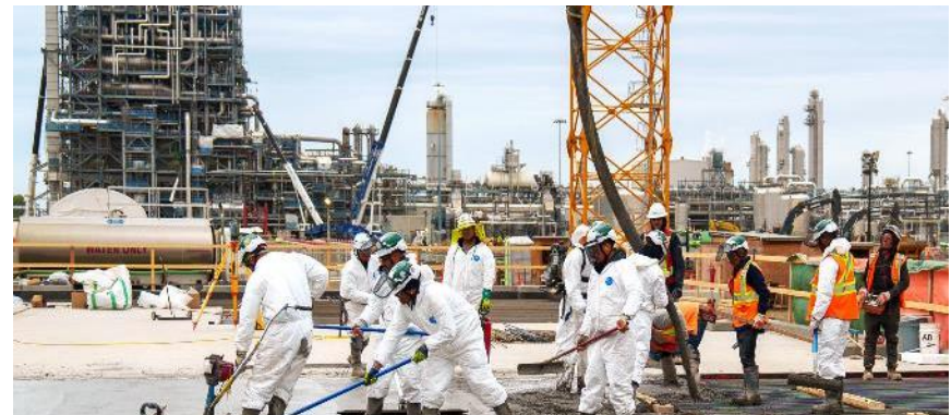
DOW FORT SASKATCHEWAN PATH2ZERO EXPANSION PROJECT // ALBERTA, CANADA
