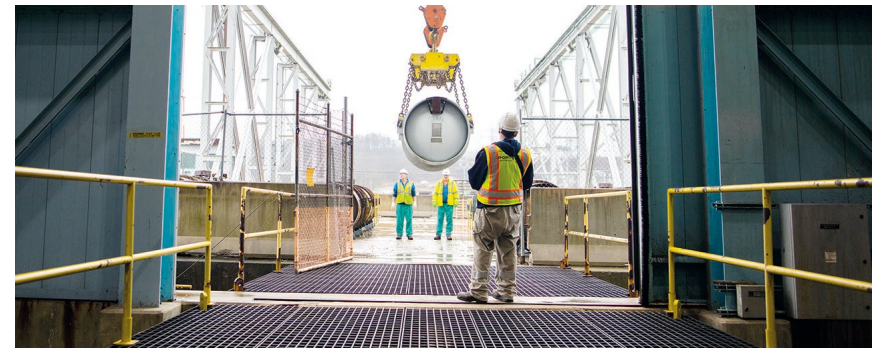
PORTSMOUTH DECONTAMINATION AND DECOMMISSIONING PROGRAM // OHIO, U.S.
