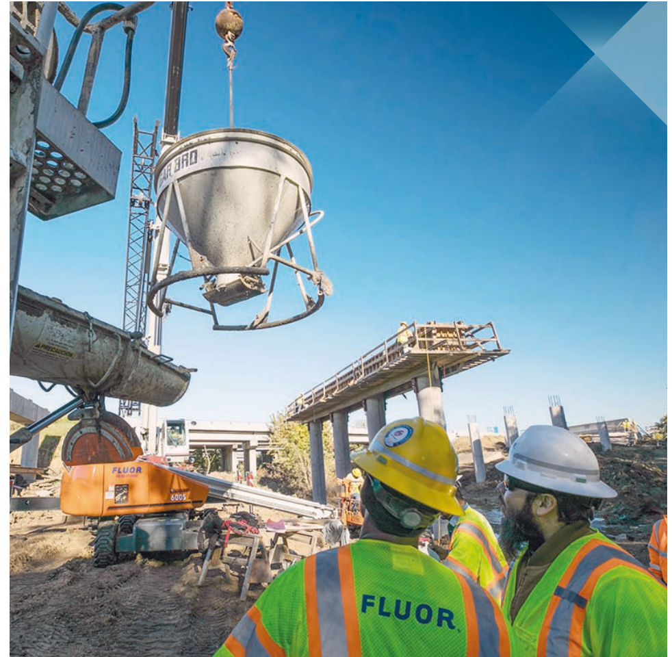
INTERSTATE HIGHWAY 20 // TEXAS, U.S.
