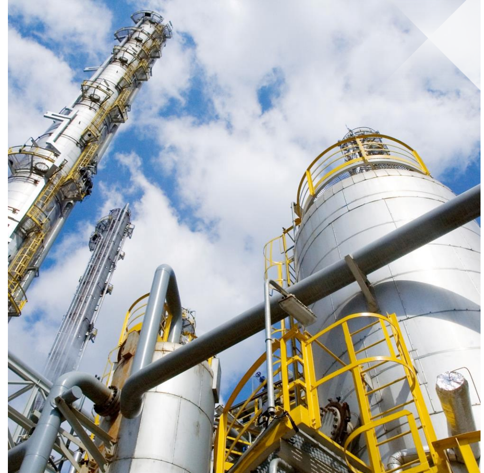
PKN ORLEN OLEFINS PLANT // PLOCK, POLAND
