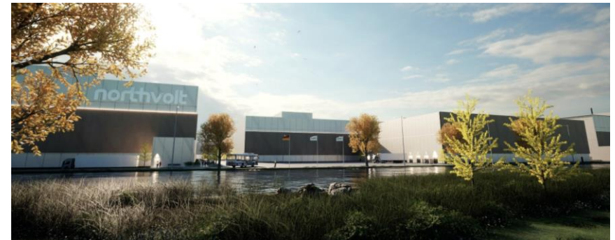
NORTHVOLT LARGE-SCALE LITHIUM-ION BATTERY FACILITY // HEIDE, GERMANY
