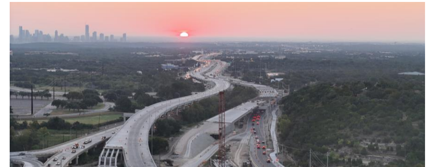
OAK HILL PARKWAY PROJECT // TEXAS, U.S.
