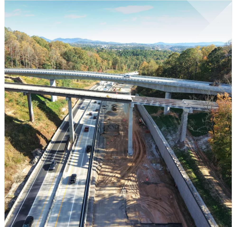
NEW BLUE RIDGE PARKWAY BRIDGE OVER I-26 // NORTH CAROLINA, U.S.
