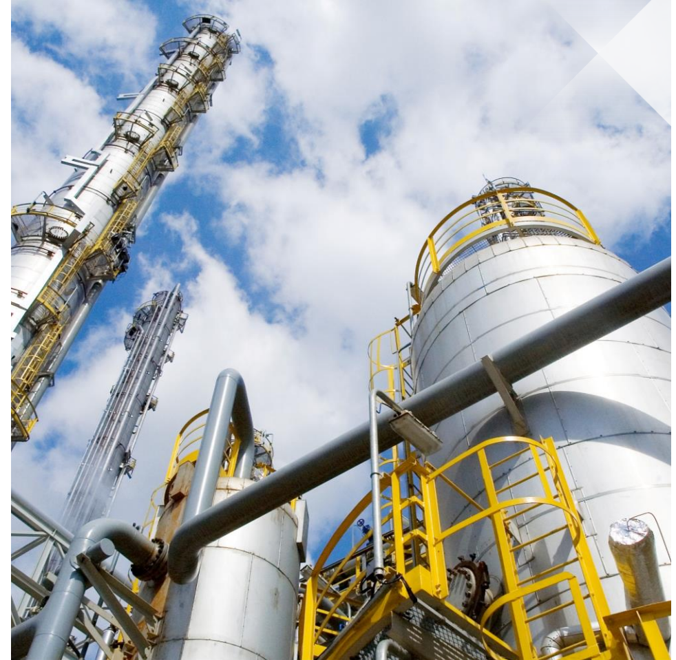
PKN ORLEN OLEFINS PLANT // PLOCK, POLAND
