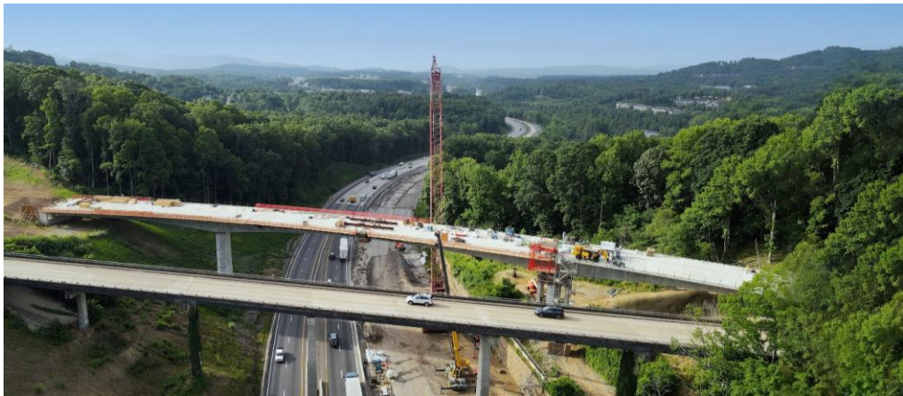
I-26 WIDENING PROJECT // NORTH CAROLINA, U.S.
