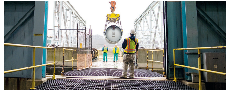
PORTSMOUTH DECONTAMINATION AND DECOMMISSIONING PROGRAM // OHIO, U.S.
