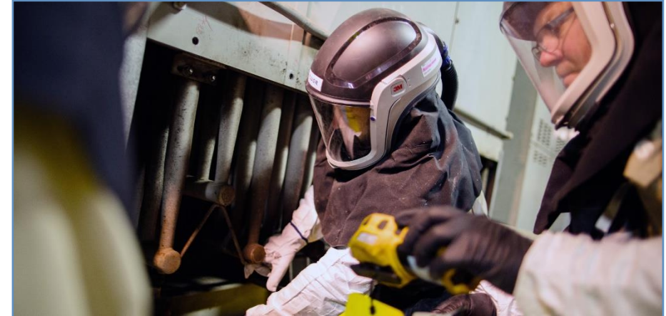
PORTSMOUTH DECONTAMINATION AND DECOMMISSIONING CONTRACT, USA
