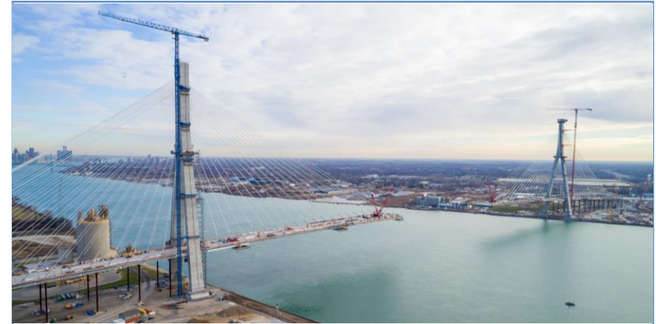
GORDIE HOWE INTERNATIONAL BRIDGE PROJECT, USA/CANADA
