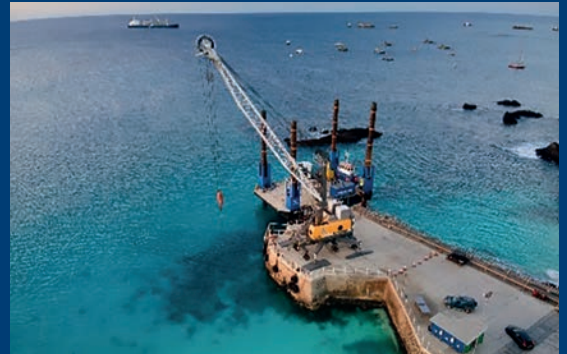
Ascension Island Airfield Rebuild // Ascension Island
