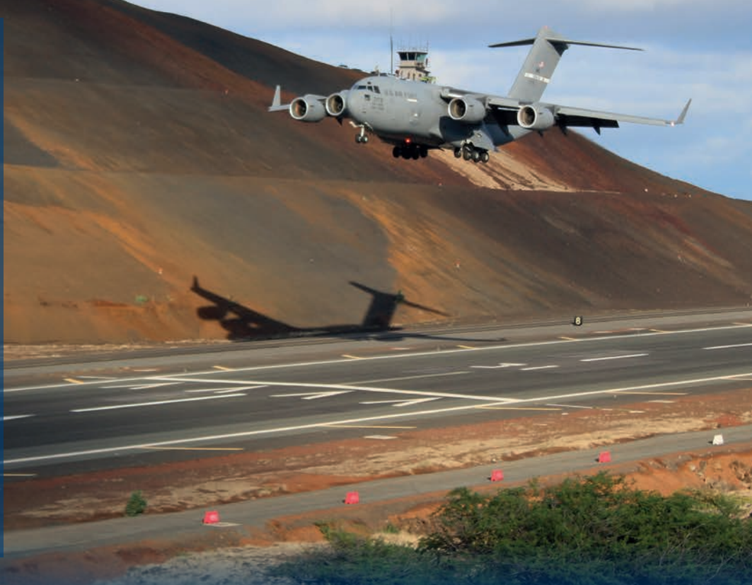
A plane lands on the rebuilt runway // Ascension Island
