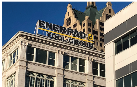
The relocation of Enerpac Tool Group's global headquarters included the renaming of the downtown Milwaukee building to the Enerpac Center
