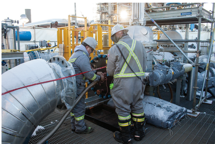
Hydratight added process and pipeline services capabilities to its offerings in 2016.
