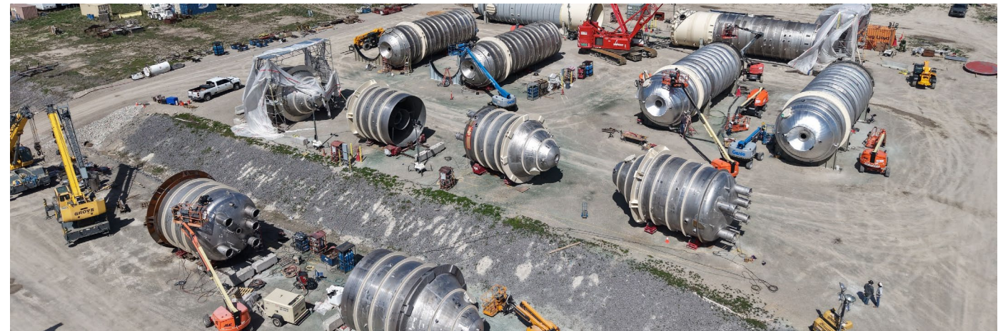
Liquid carbonate crystallizers are being assembled at Great Basin Industrial in Utah
