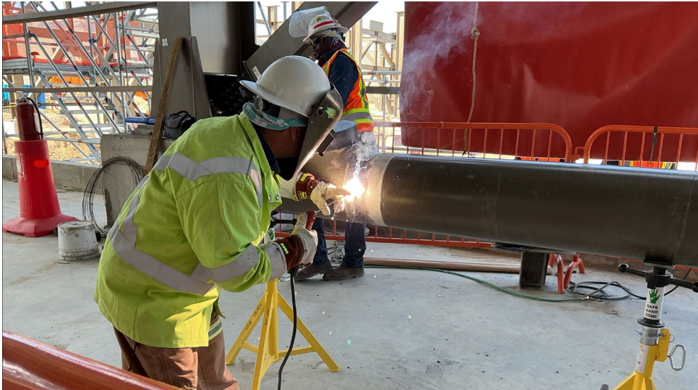
The first weld of an aboveground pipe at the Filtration Building
