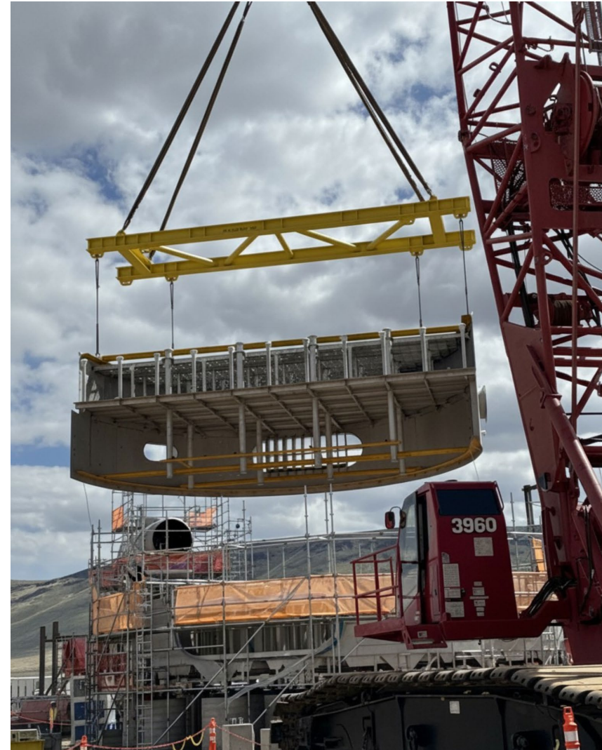
Installation of the second floor at the sulfuric acid plant
