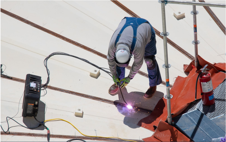
The first seal weld on a CCD thickener
