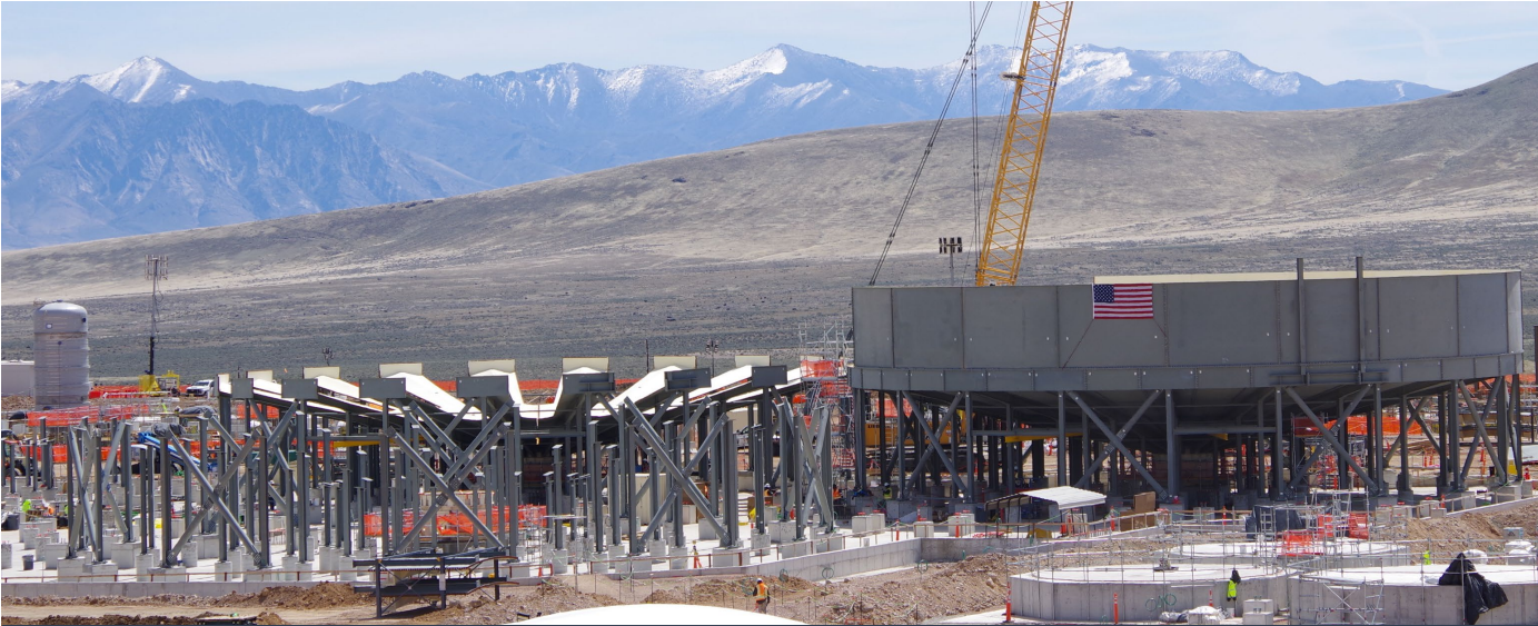
The buildout of eight counter-current decantation (CCD) units continue
