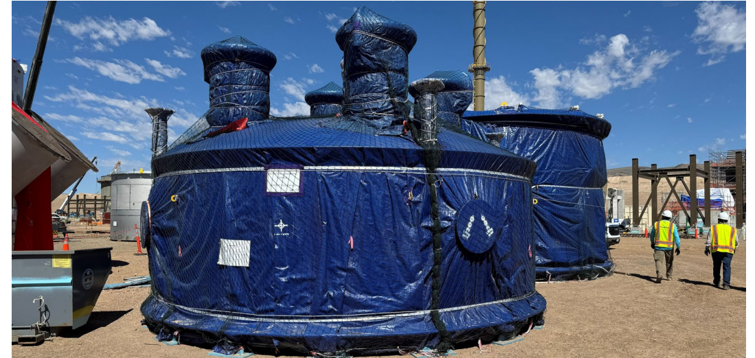
Components of the Sulfuric Acid Plant's Inter-pass Absorption Tower arriving at site
