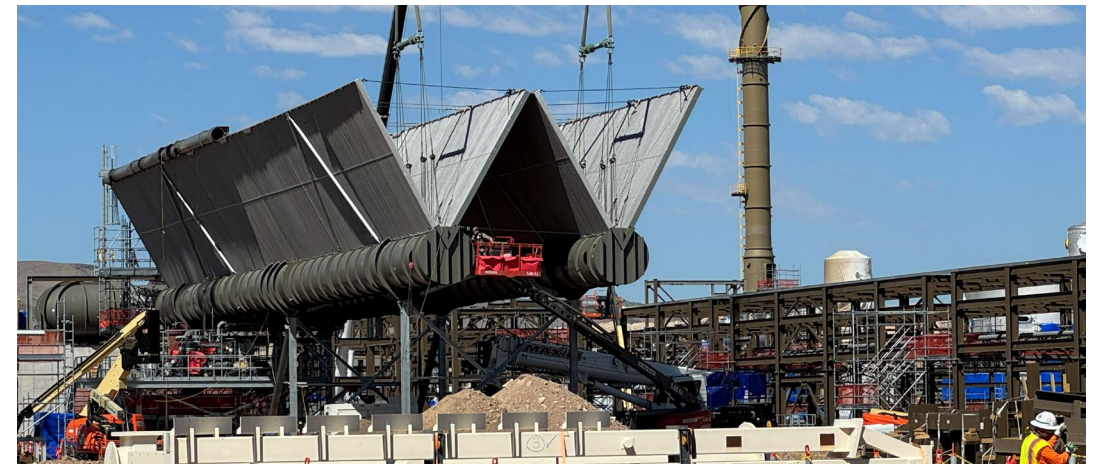
W heat exchanger bundle installed on the Air Cooled Condenser
