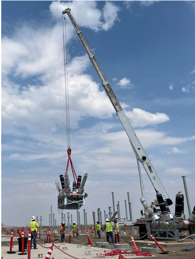
One of three high voltage circuit breakers has been installed
