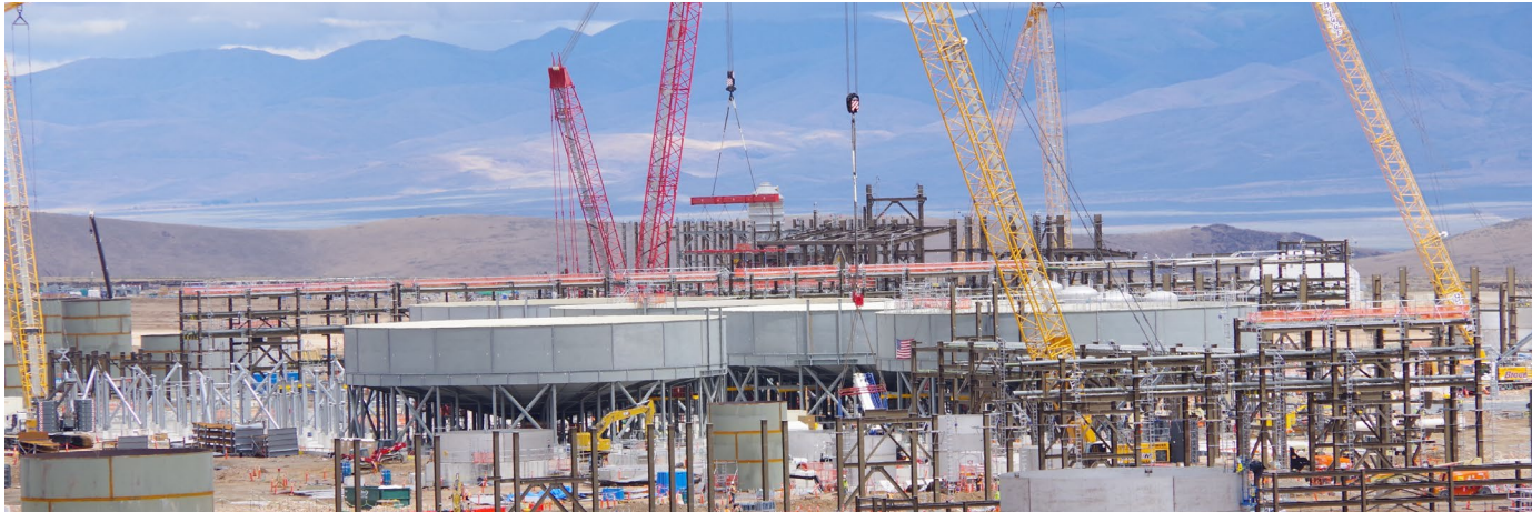
Progress continues on the eight counter-current decantation thickener tanks
