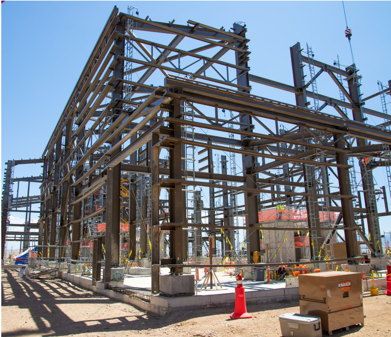
Progress at the Magnesium Sulfate building
