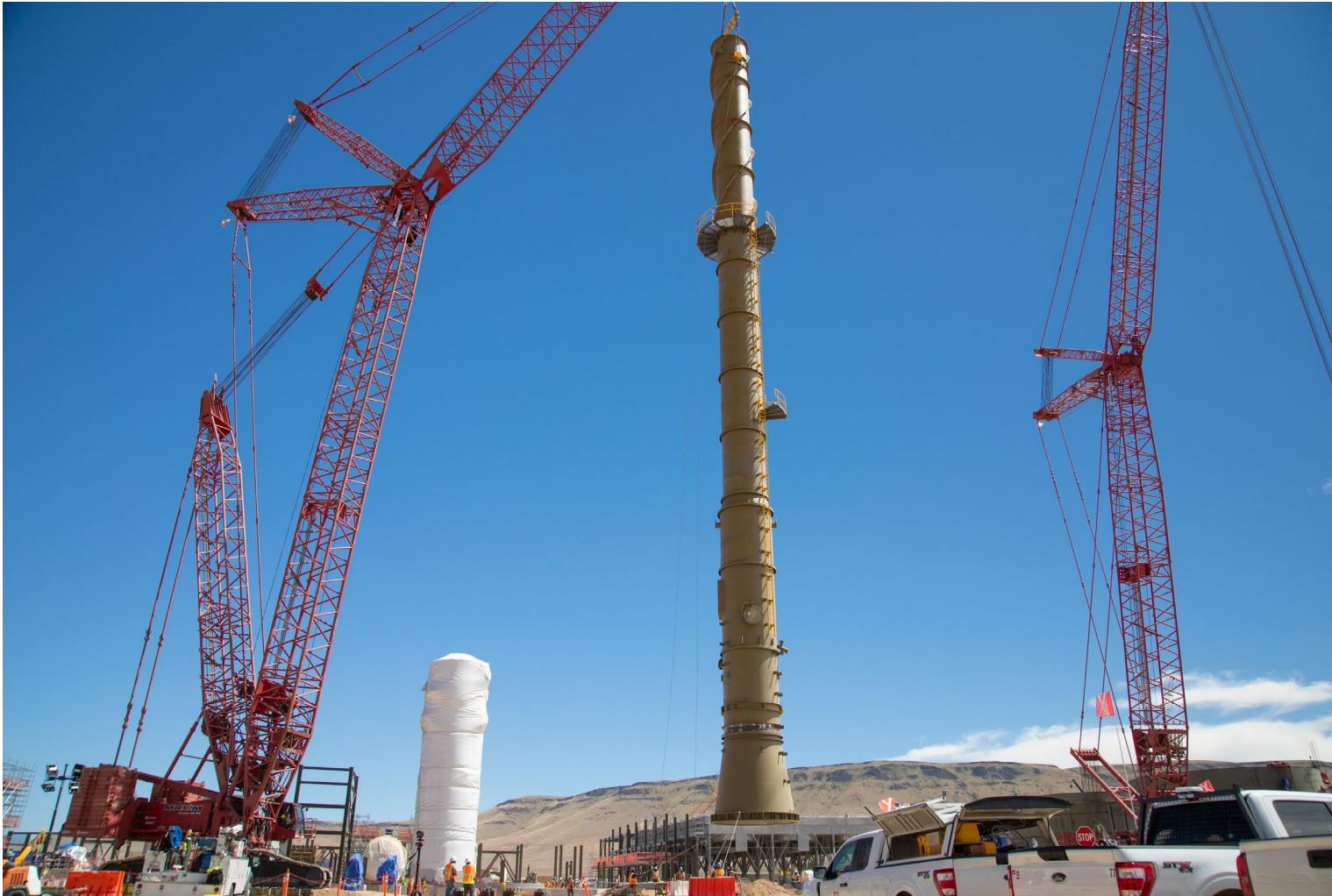
The 198-foot Duplex Plant Stack for the Sulfuric Plant
