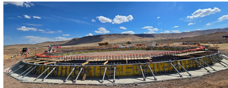
Foundation for one of two liquid sulfur tanks
