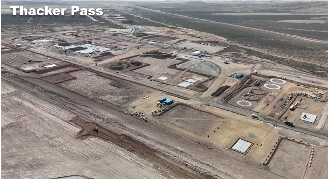
Aerial of Thacker Pass processing plant area
