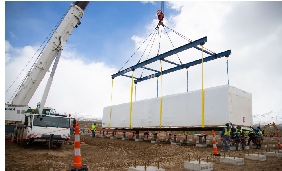
First module housing unit installed in mid-March 2025
