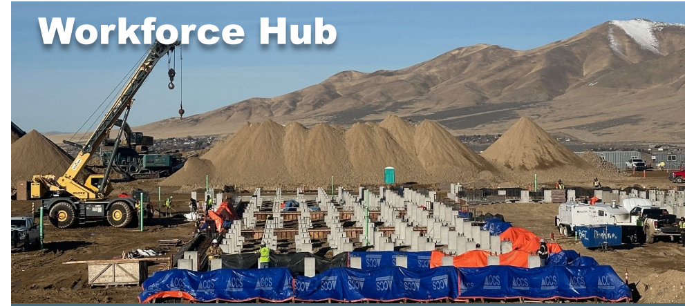
Over 380 pre-cast foundations have been installed; first occupancy expected in H2 2025
