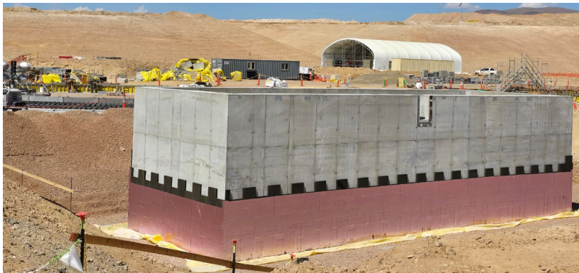
Insulation installation at the Liquid Sulfur Pit
