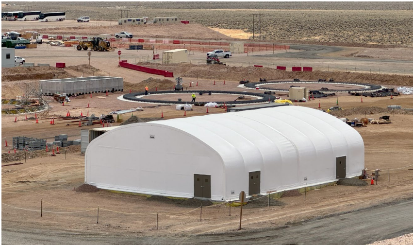
One of the completed break tents at Thacker Pass, there will be six in total
