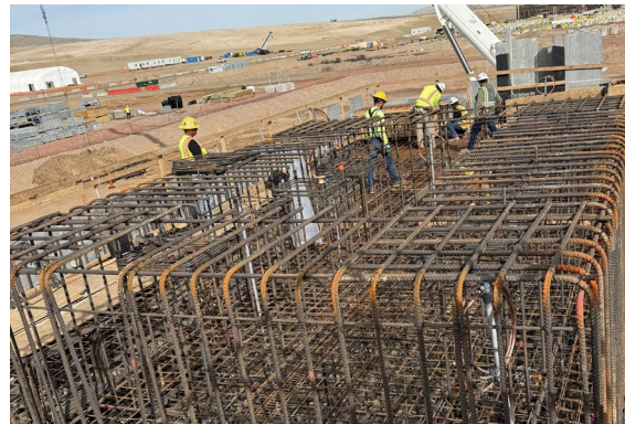
Foundation prep for the Steam Turbine Generator
