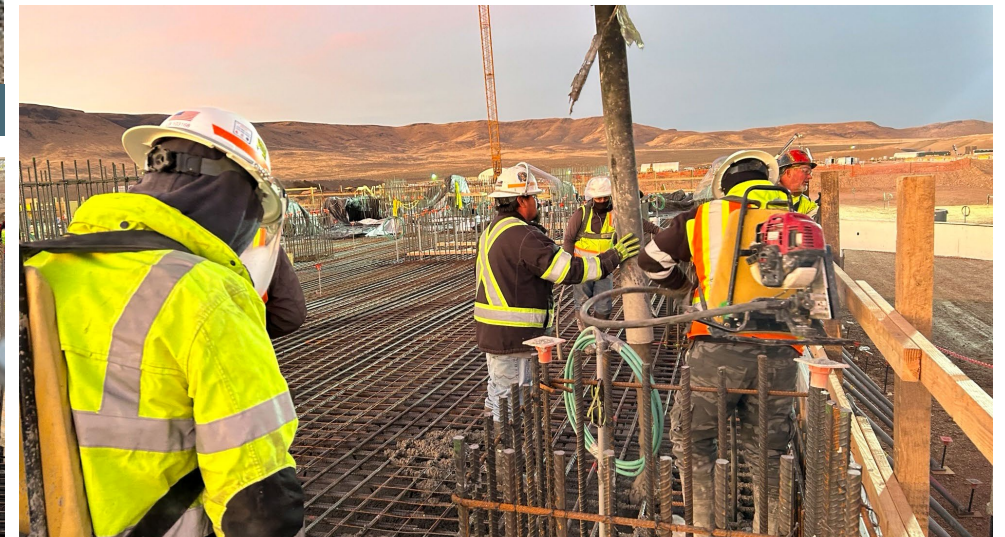
Concrete pour at the Run of Mine thickener area
