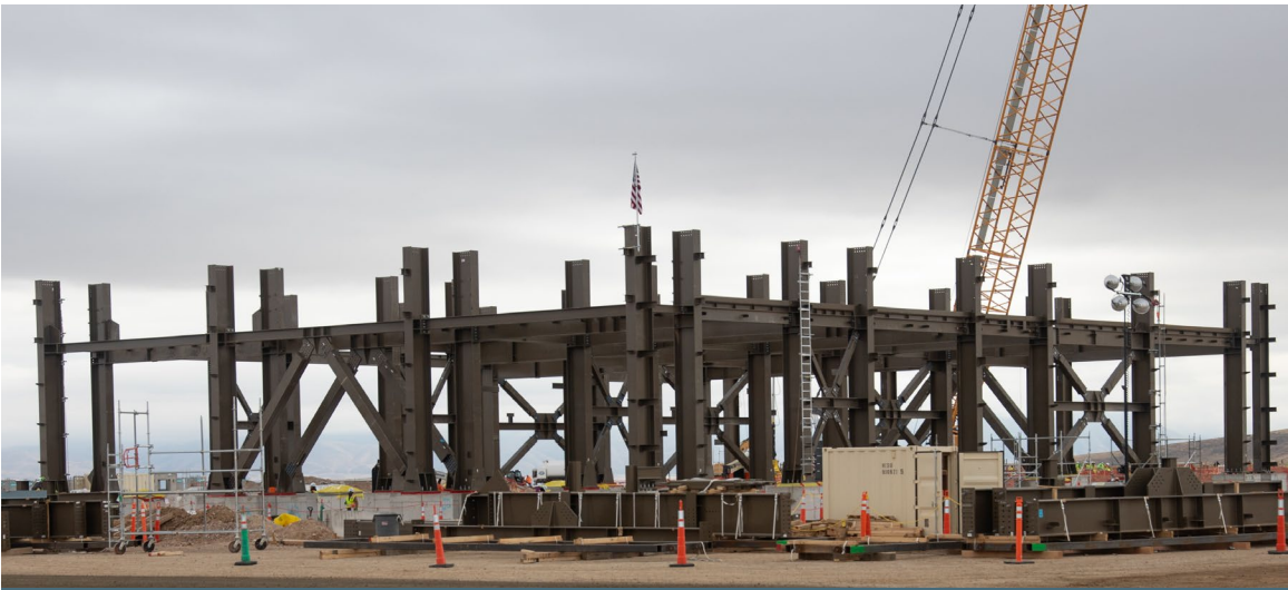
Progress at the Filtration Building
