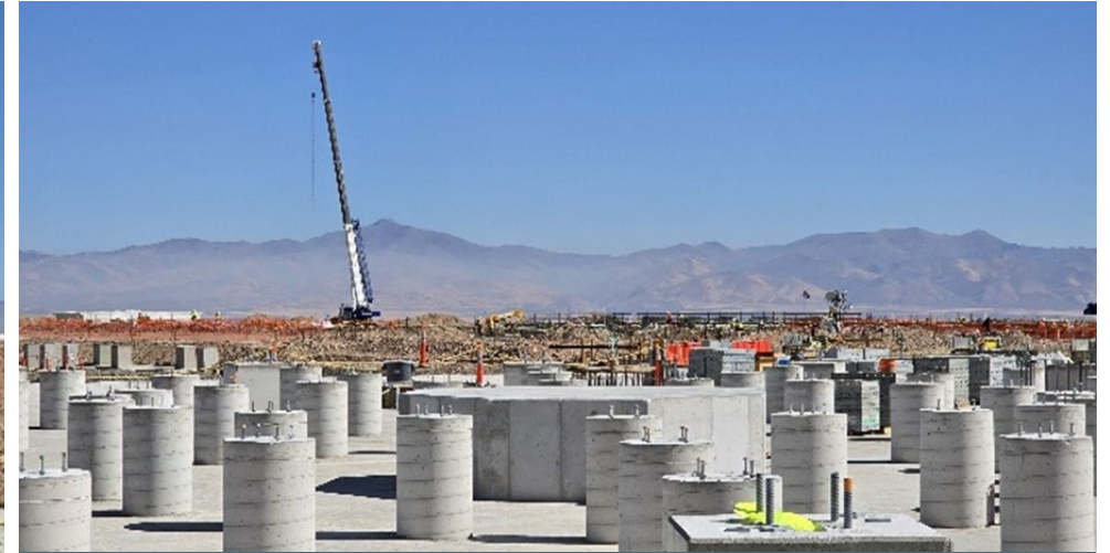
Completed central pedestals for the CCD Thickener
