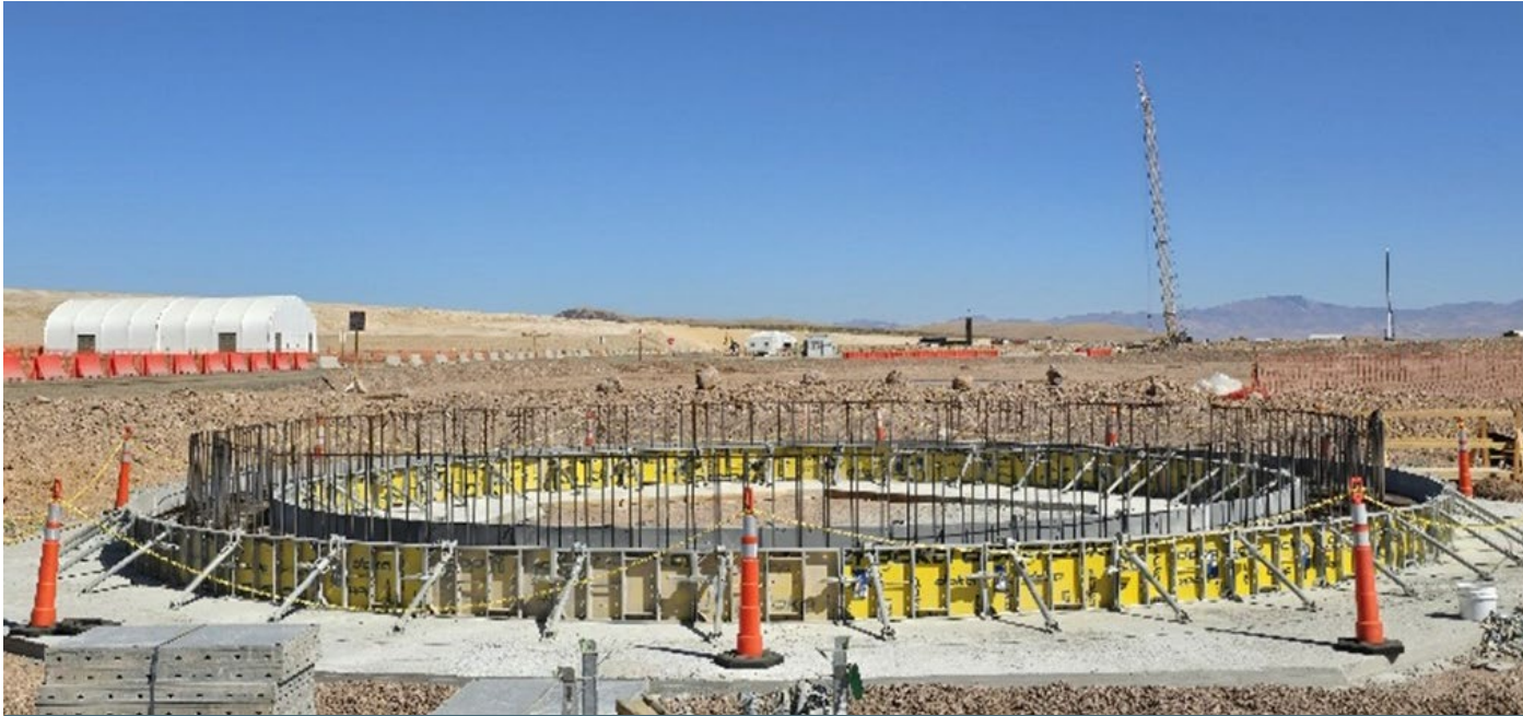
Rebar installation ring at the Treated Water Tank
