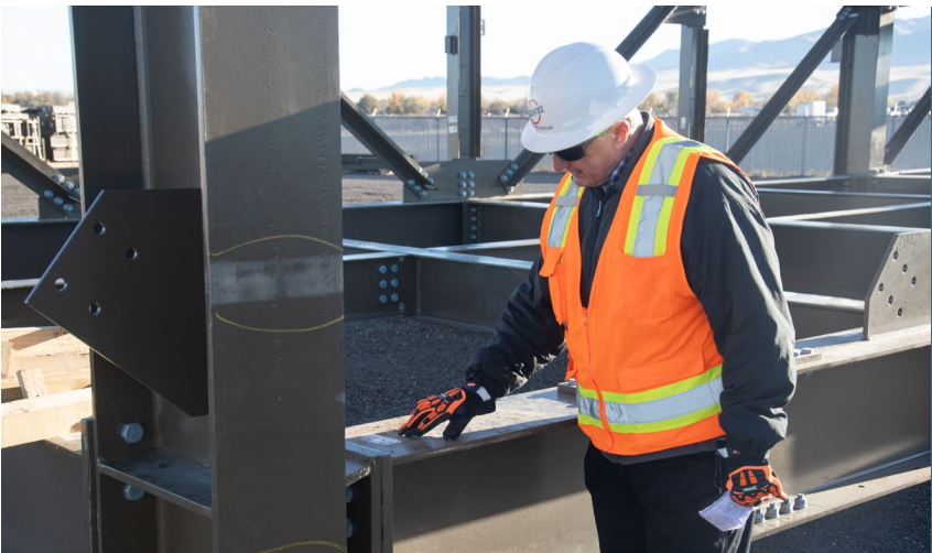
A Bechtel worker inspects one of the labels that identifies each piece of steel
