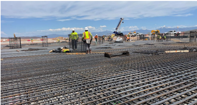
First permanent concrete pour on the process plant pad in May 2025; (below) rebar installation
