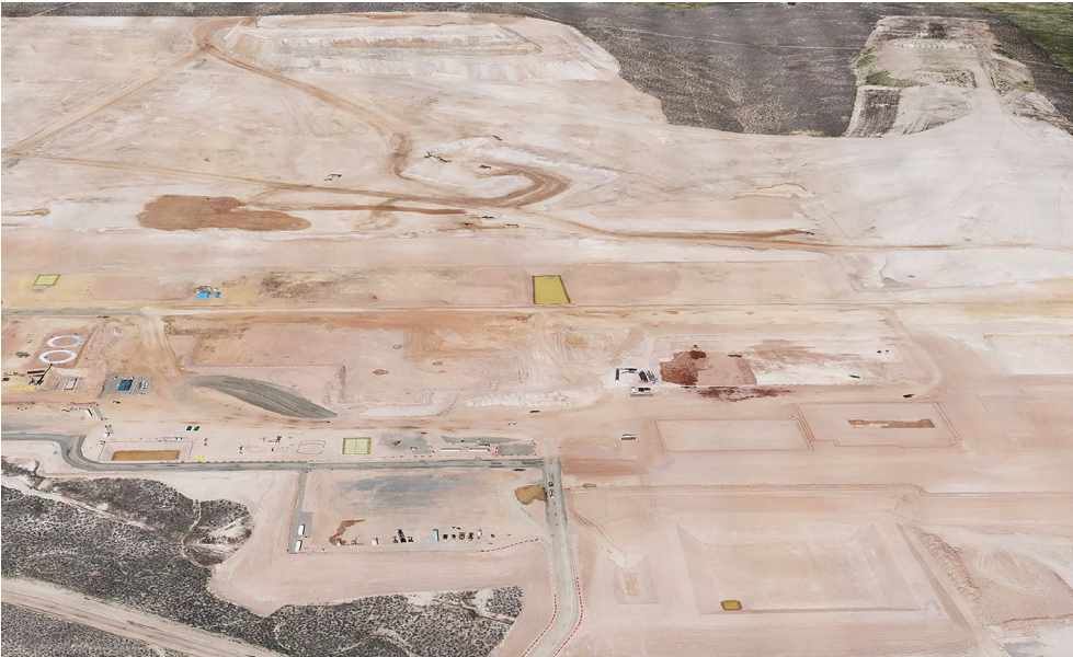
Aerial view of the process plant pad as of May 2025
