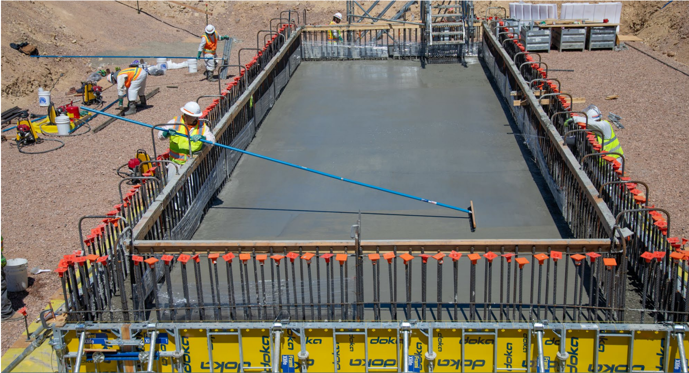
First permanent concrete pour on the process plant pad in May 2025; (below) rebar installation
