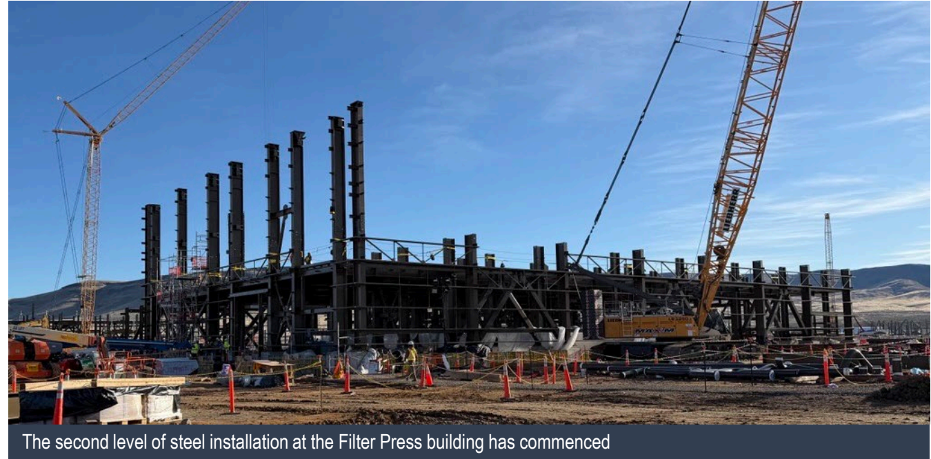
East-west pipe rack supports on the left, and the Magnesium Sulfate building in the background
