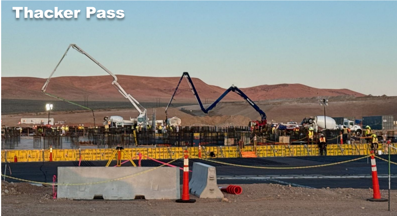
Two concrete pump trucks operate simultaneously to enhance efficiency and reduce overall pour time in the CCD area
