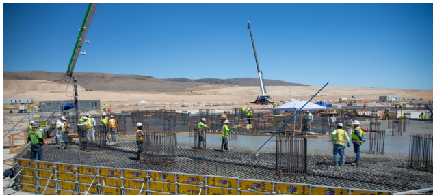
Concrete placements for the CCD area
