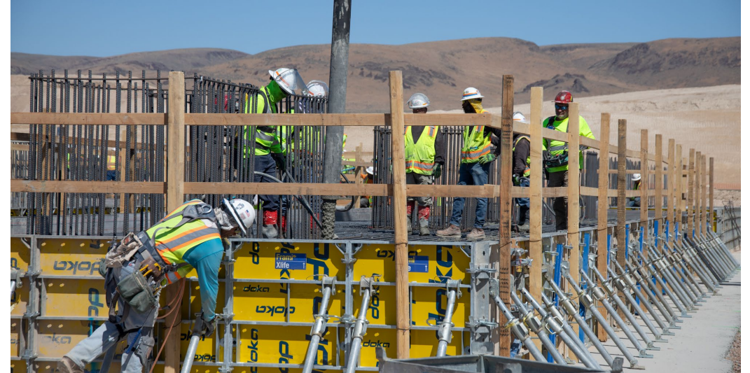
Foundation placement for the Magnesium Precipitation Filtration Building
