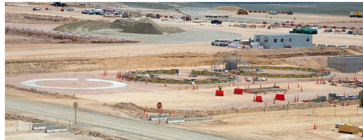
Sulfur tank foundations (the circles) are starting to take shape
