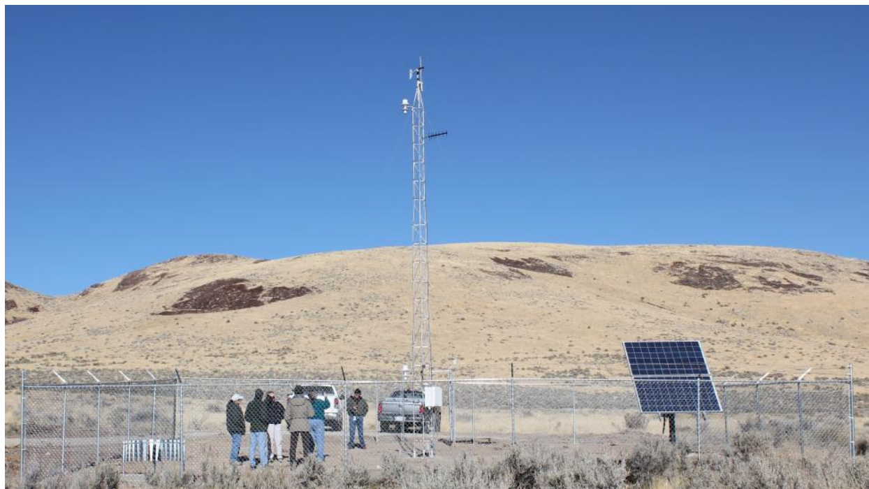
Figure 4-1 On-Site Meteorological Station, Including Tower, Solar Power Station, and Security Fence
