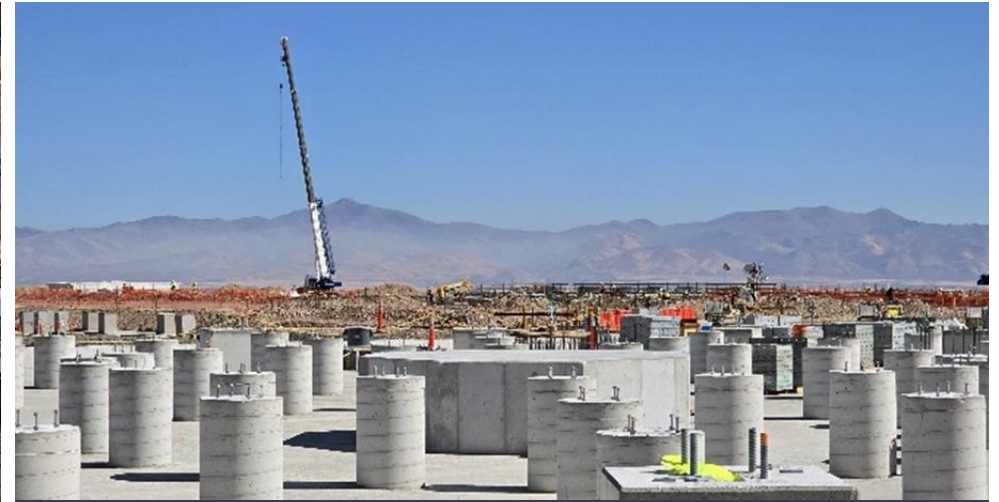
Completed central pedestals for the CCD Thickener
