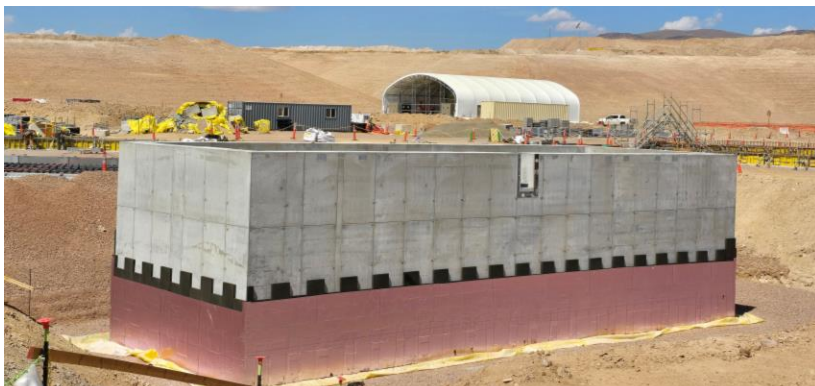
Insulation installation at the Liquid Sulfur Pit
