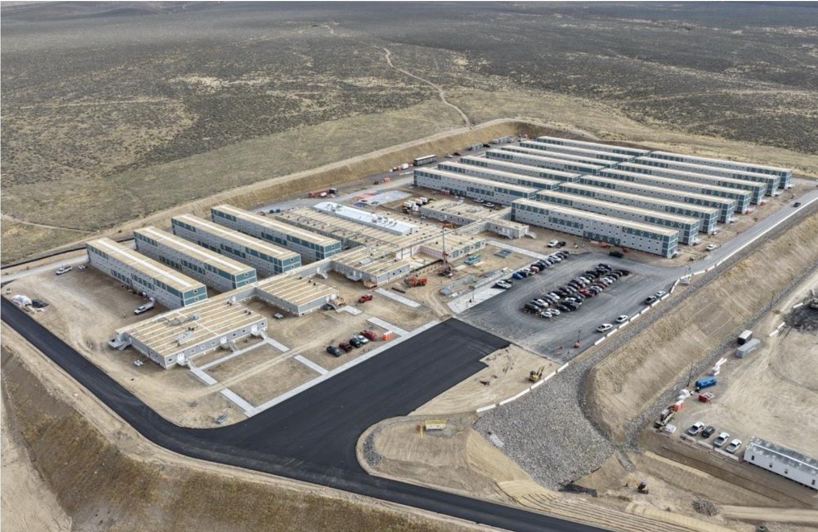
The Workforce Hub is completed and welcoming residents in phases
