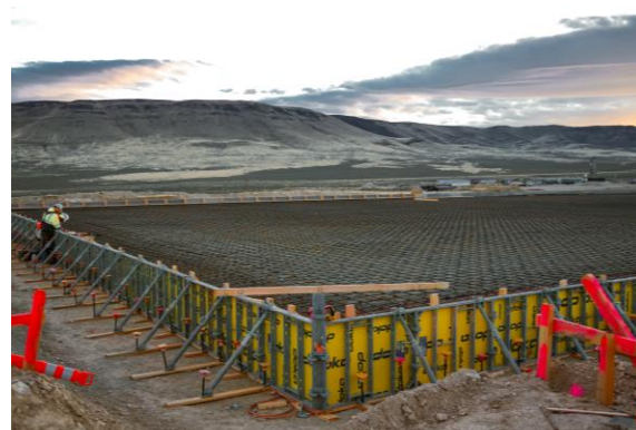
Foundation work for the site temporary warehouse
