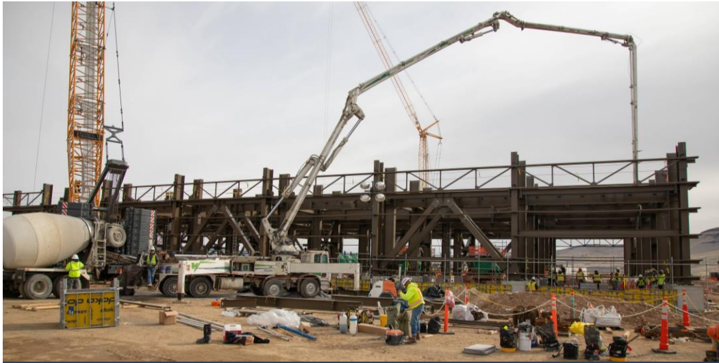
Pouring the concrete floor at the Filtration Building
