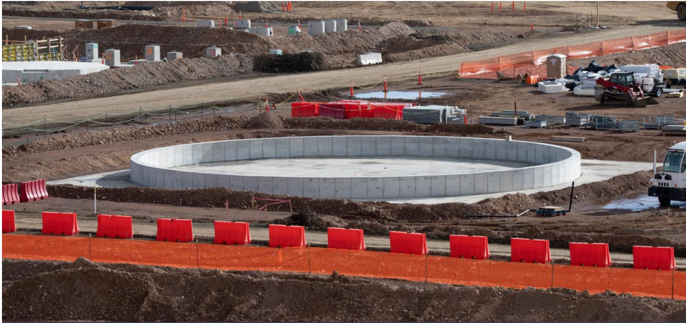
A large, tank foundation in the Water Systems area
