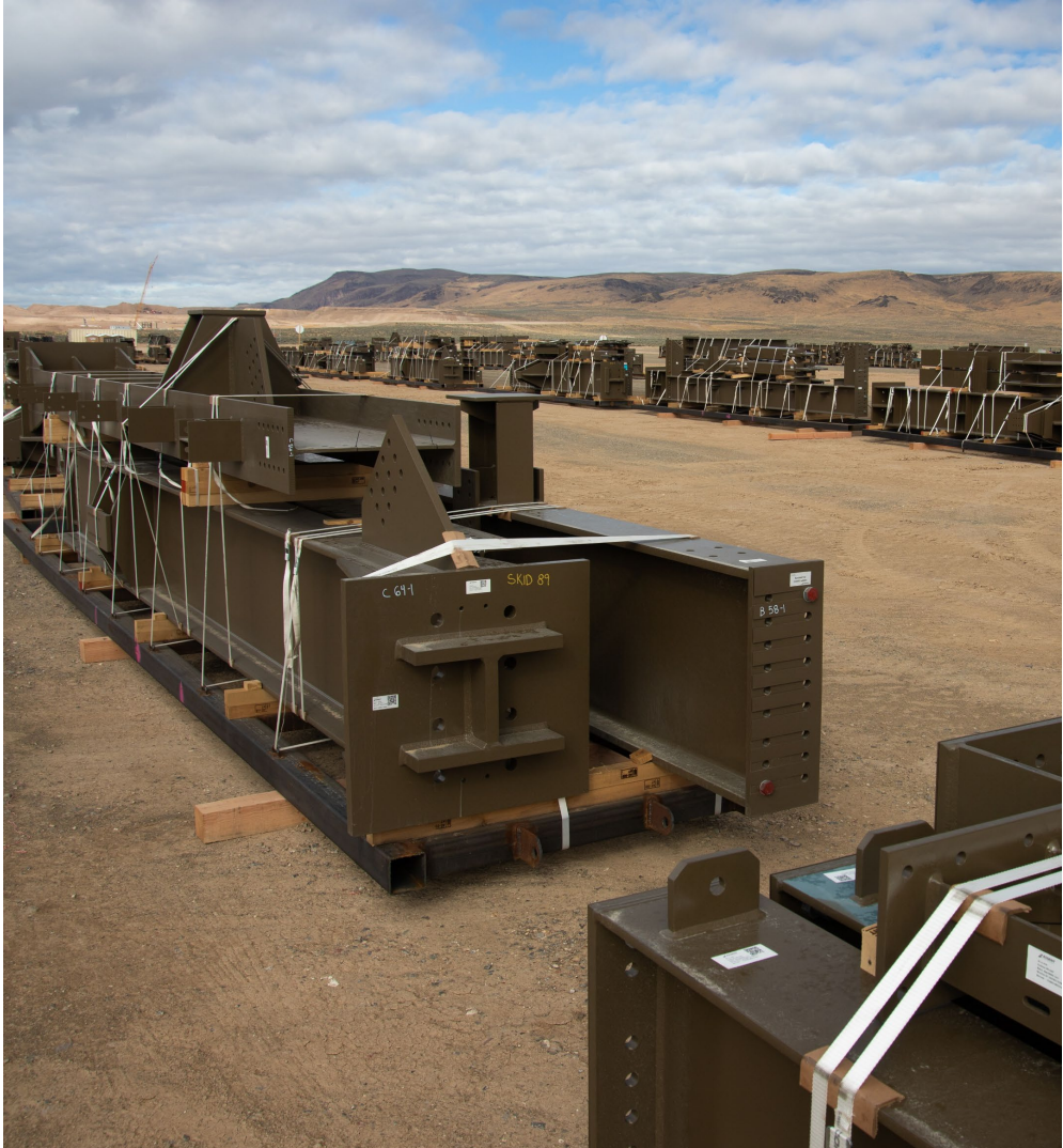
Steel awaiting installation at the Thacker Pass laydown yard
