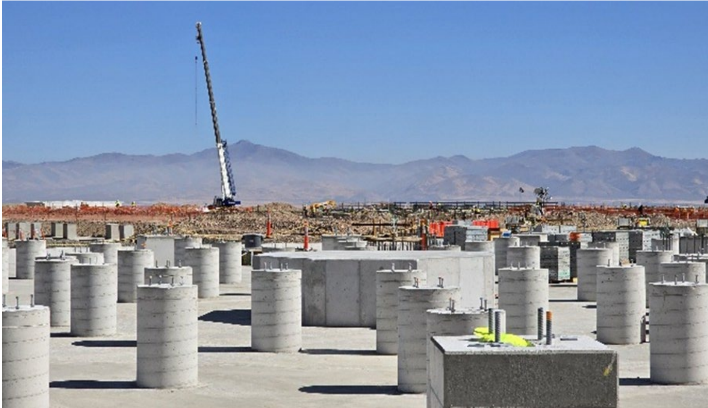
Completed central pedestals for the CCD Thickener
