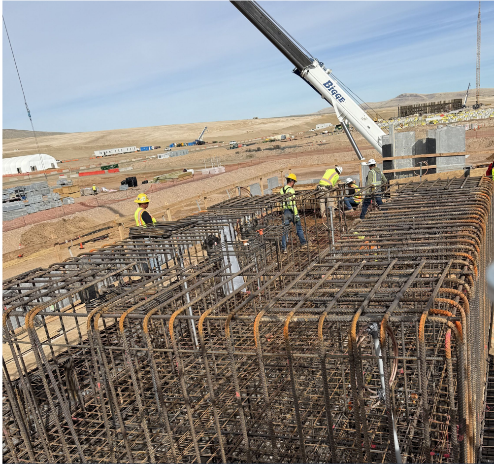
Foundation prep for the Steam Turbine Generator
