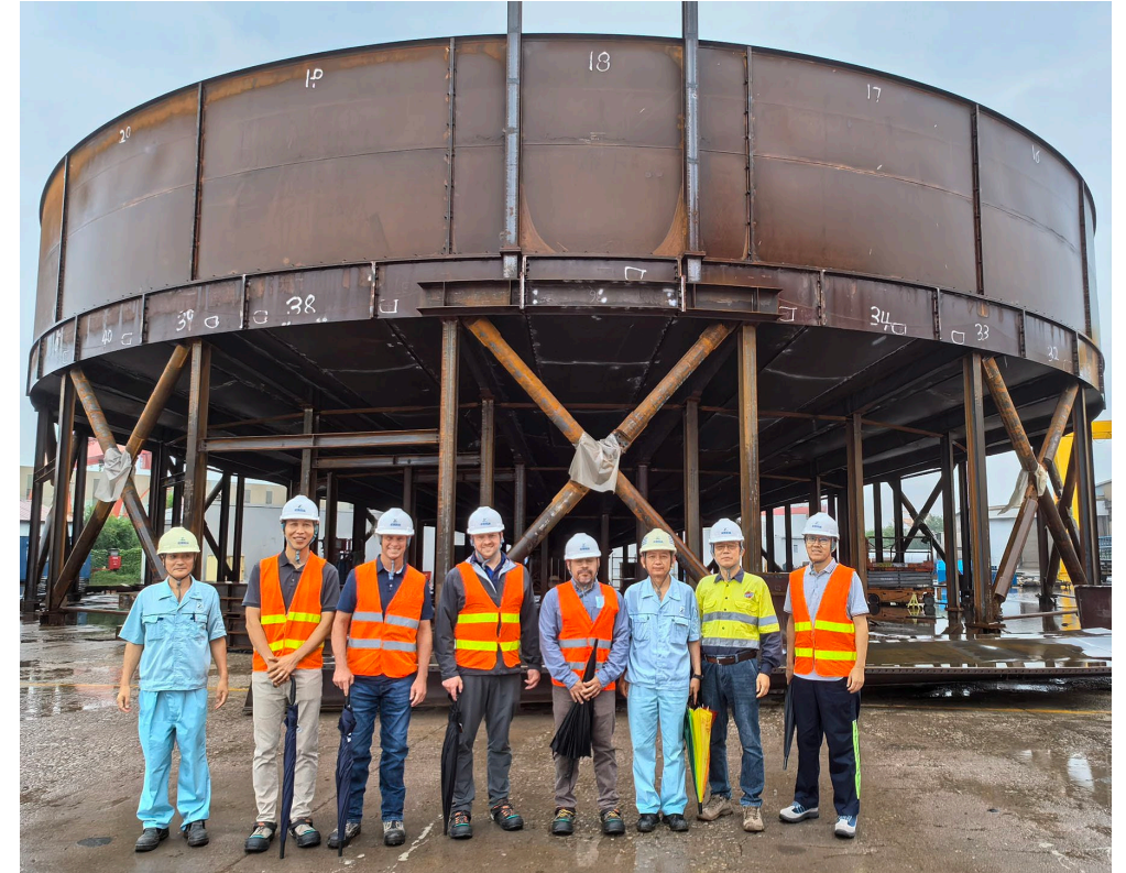
CCD Thickener trial assembly
