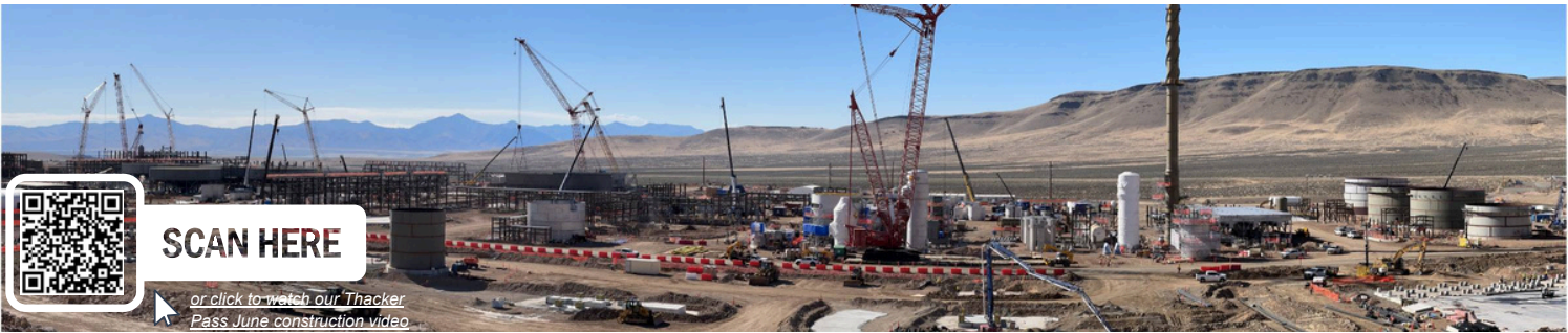
A panoramic view of the Thacker Pass construction site as of early July 2026. More than 15 cranes are now in operation. Check out our latest construction video on YouTube.
