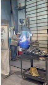
A CarWil technician is pictured in the their Winnemucca headquarters, welding part of a pre-assembled module component for installation at Thacker Pass.
