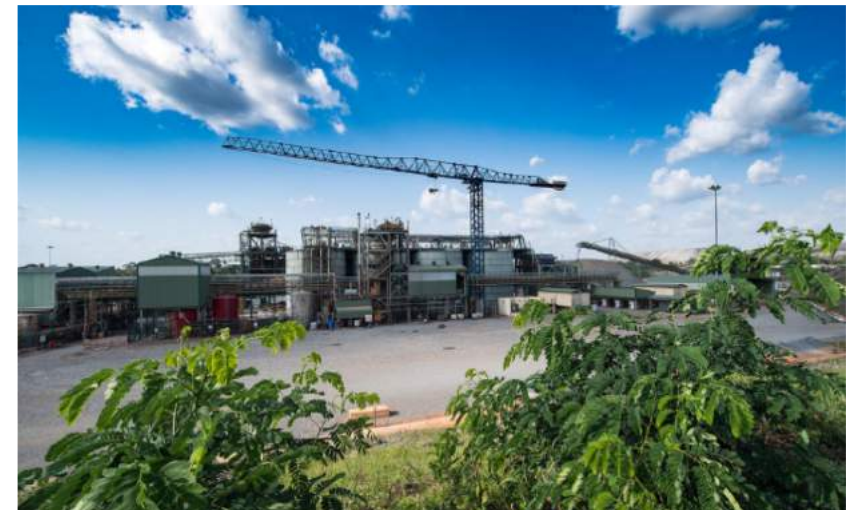
Upgraded 5Mtpa Plant
