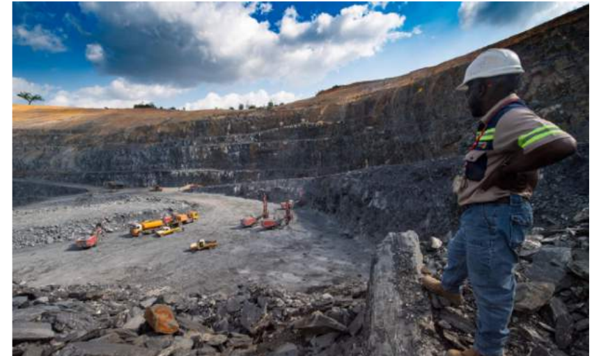
Current Progress of Cut 2 Pushback
