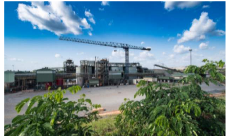
Upgraded 5Mtpa Plant
