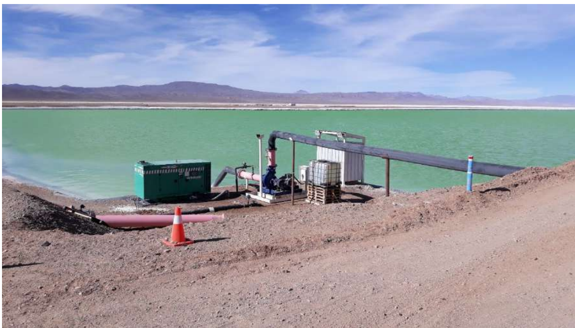
Figure 17.6 Evaporation Ponds – Transfer Pump Station
