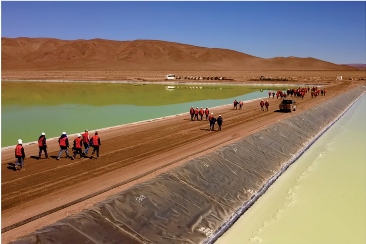
Figure 17.2 Evaporation Ponds at Cauchari Salar
