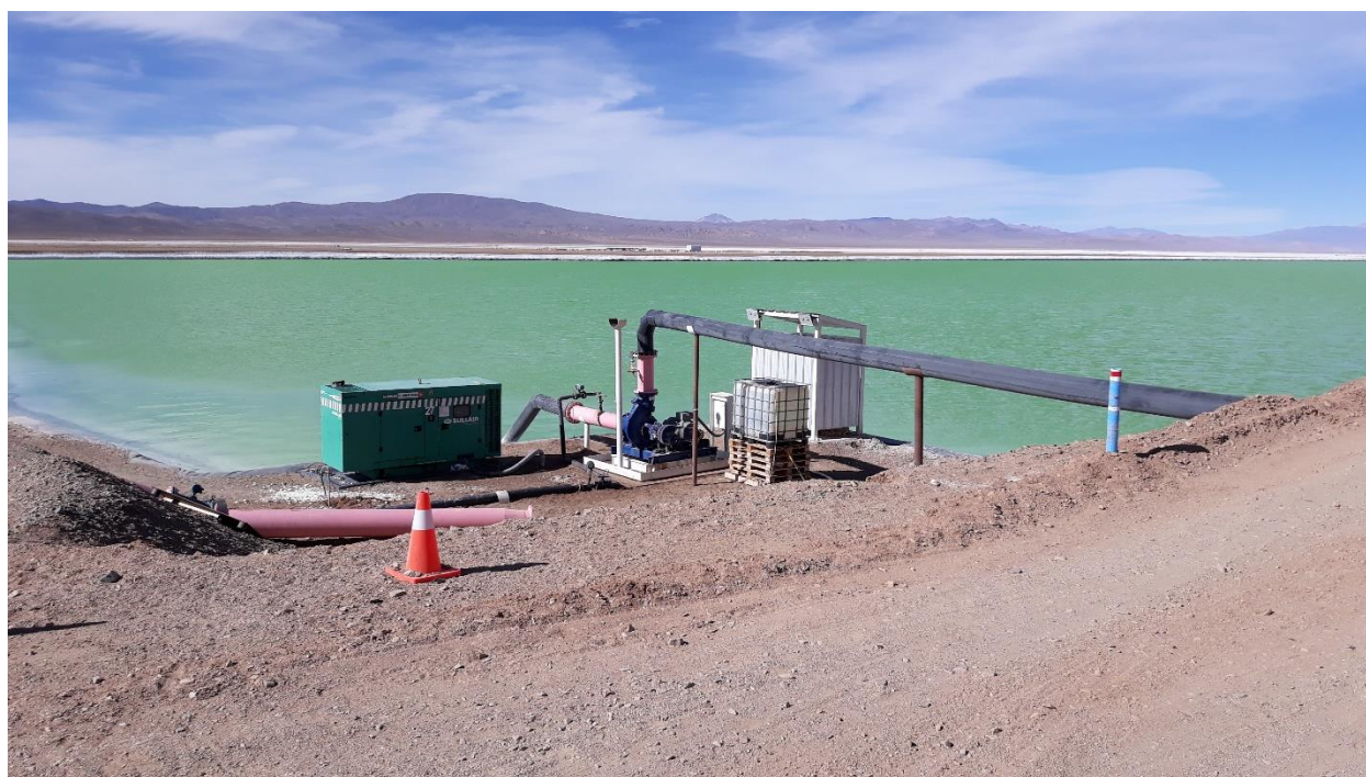
Figure 17.6 Evaporation Ponds – Transfer Pump Station
