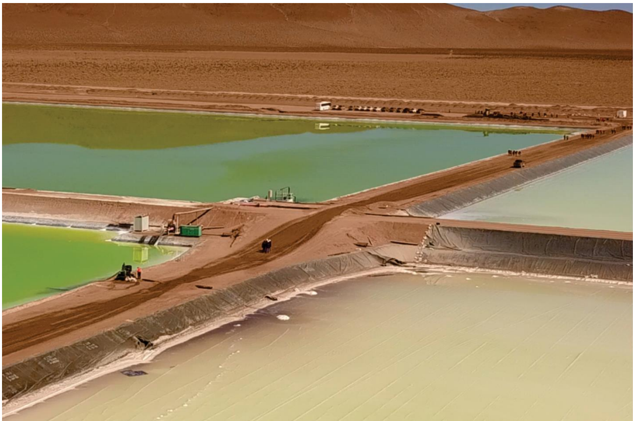
Figure 17.4 Evaporation Ponds
