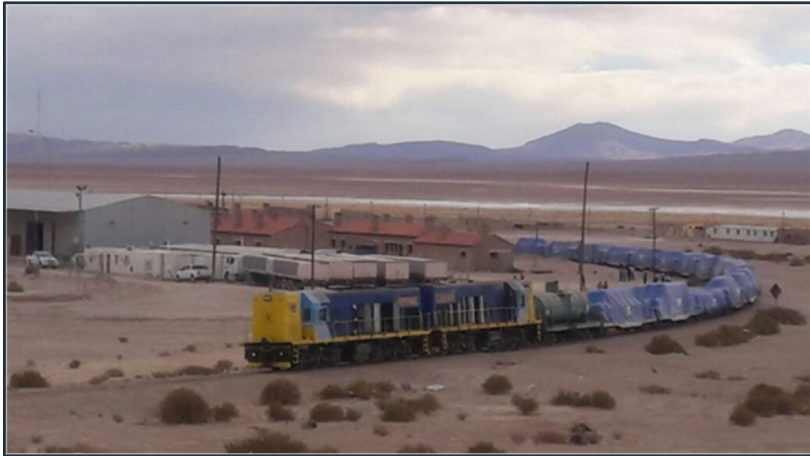
Figure 15-6. Livent Salar de Pocitos Railway Station
