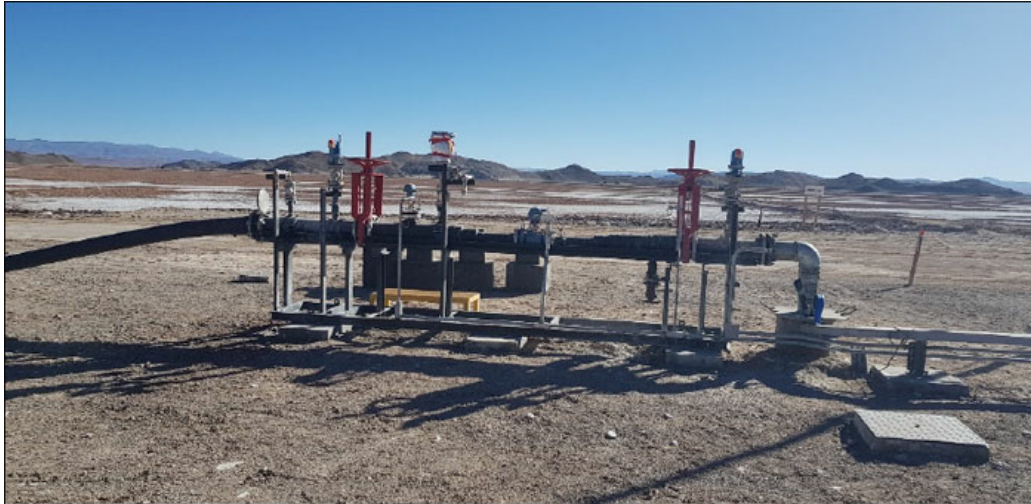
Figure 13-2 - Production Well SVWP21-02.
