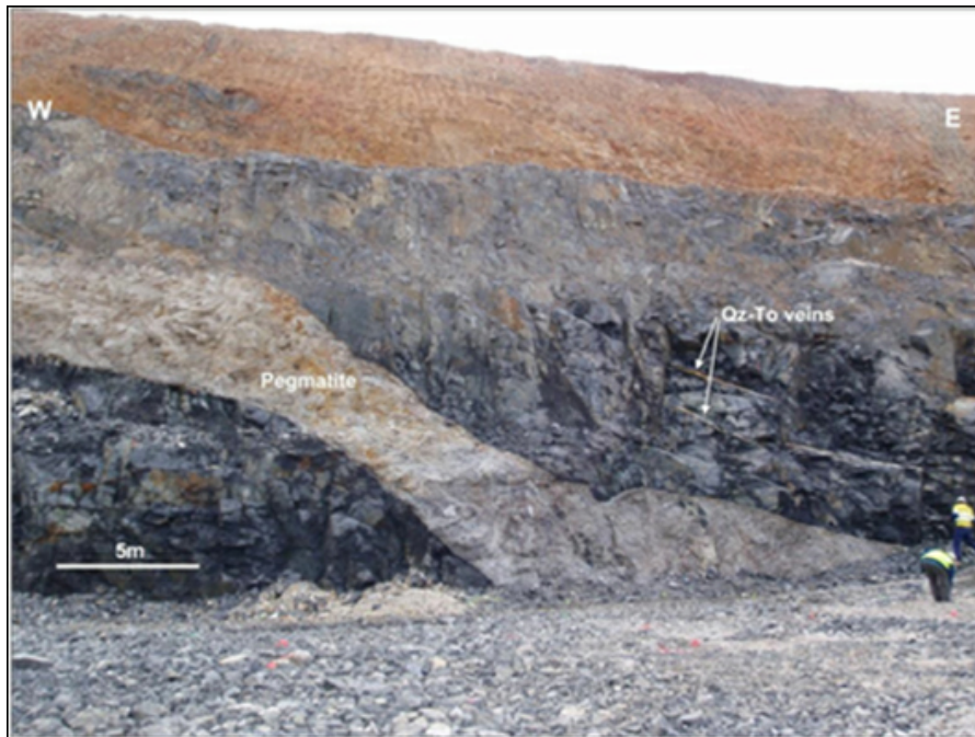
Figure 6-7 - Mt Cattlin Pit 1A north wall showing pegmatite and quartz tourmaline veins.
