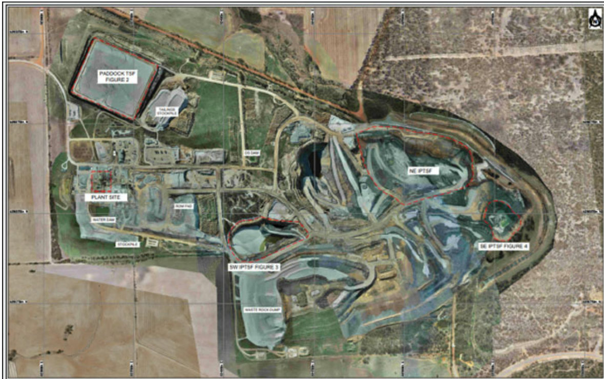
Figure 15-2 - Tailings Storage Facilities.
