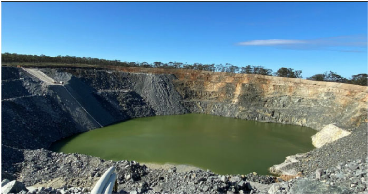
Figure 15-6 - SE IPTSF Decant Pond and Return Water System (October 2022).
