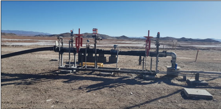
Figure 13-1 - Production Well SVWP21-02.
