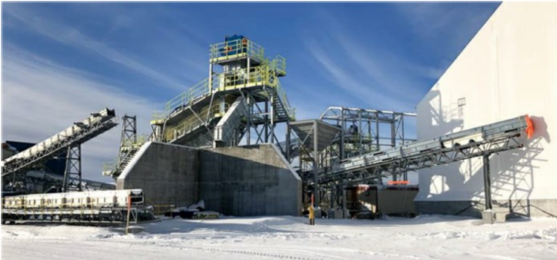
Figure 21-2 View of Screening Tower and Concentrator
