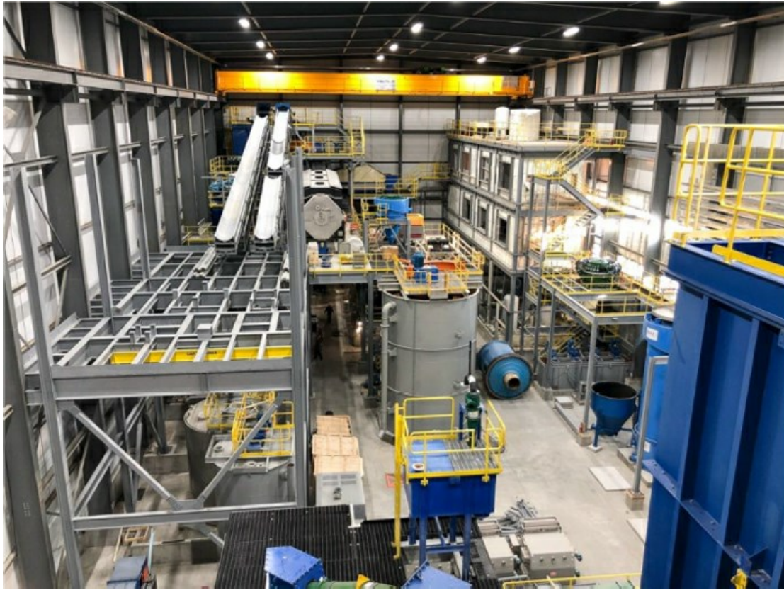
Figure 21-3 View of Concentrator Interior
