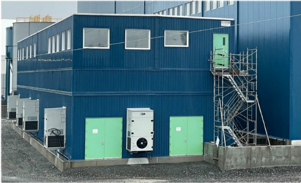
Figure 21-11 Concentrator Main Electrical Room, Offices and Laboratory
