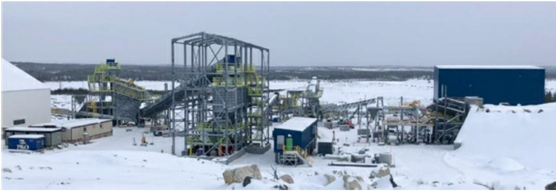
Figure 21-1 View of Primary and Cone Crusher Buildings
