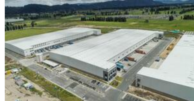
Logistic Park Calle 80, Bogota, Colombia
