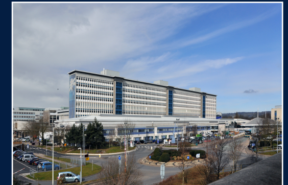
University Hospital Wales Cardiff, United Kingdom
