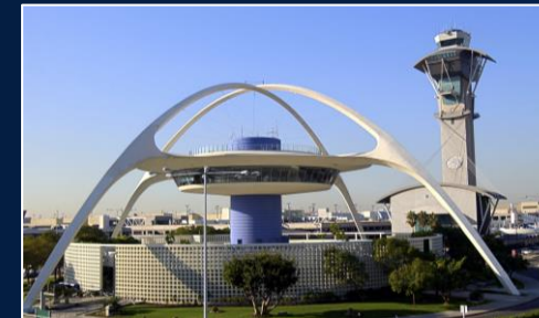
Terminal 4 at LAX Los Angeles, California
