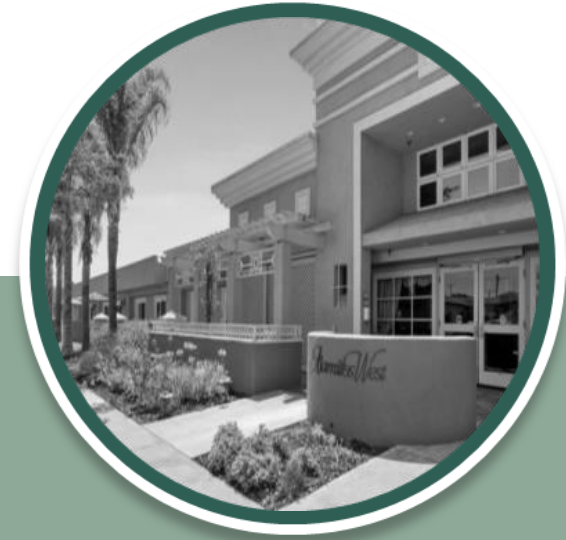
Alamitos West Health & Rehabilitation California
