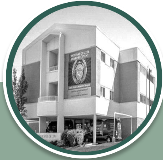
South Davis Community Hospital Utah
